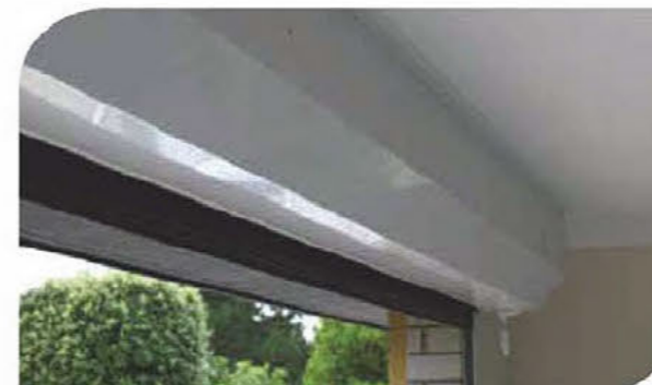
Internal view showing canopy (box)
